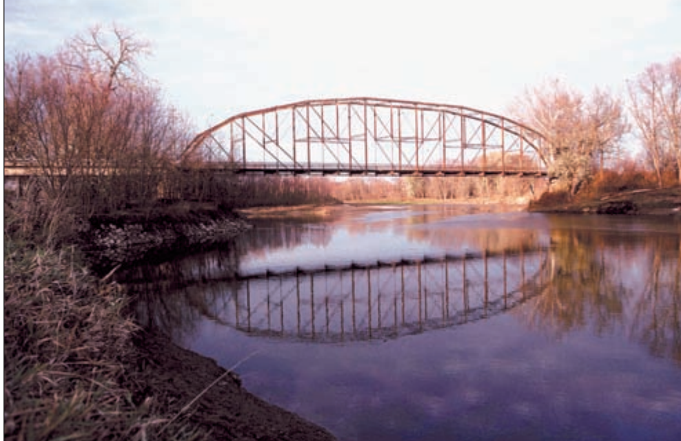
This 1895 iron structure, now dismantled, will find a new home in Delphi
