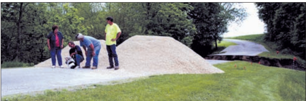
Stone barriers for safety
