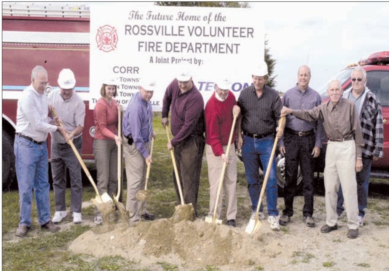
A groundbreaking ceremony was held last week for a new fire station for the Rossville Volunteer Fire Department. Pictured l-r are: Jerry Frey, Clay Township advisory board; Wayne Remaly, Clay Township advisory board; Marla Milazzo, Clay Township trustee; Allen Remaly, Rossville Town Council president; Matt Marley, Ross Township trustee; Rick Ryan, Owen Township trustee; Lewis Flohr, Owen Township advisory board; Dan Lahrman, Ross Township advisory board; Carl Seest, Ross Township advisory board; Jim Unger, Owen Township advisory board. Tecton of Lafayette is the construction manager. Comet photo by Jennifer Archibald
