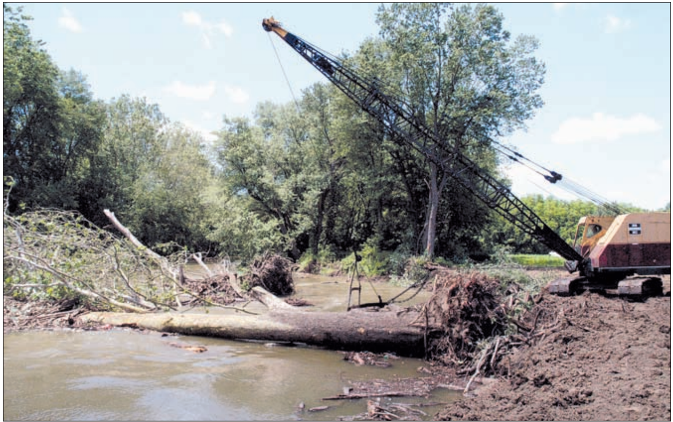
A log jam on Wildcat Creek at the north edge of Burlington is finally getting the attention it deserves. Town officials have been working for several months trying to find a way to remove the debris. Their concern was potential damage to the town's sewage treatment plant due to the backed up creek. A month ago Stacy Flick from the Indiana Department of Transportation's LaPorte District was given orders to take care of the problem. He said it took a few weeks to get the proper permits and to bid the project out before starting Monday. Shepherd's Excavating of Winamac was awarded the bid. Typically, INDOT is only concerned with property in and around the bridge, said Flick, who is the project supervisor. This problem is down from the bridge, however it has the potential of affecting the bridge if it is not removed. INDOT is "doing it to be a good neighbor," Flick said. "We hope to have this done this week. The water has already dropped quite a bit." Comet photo
