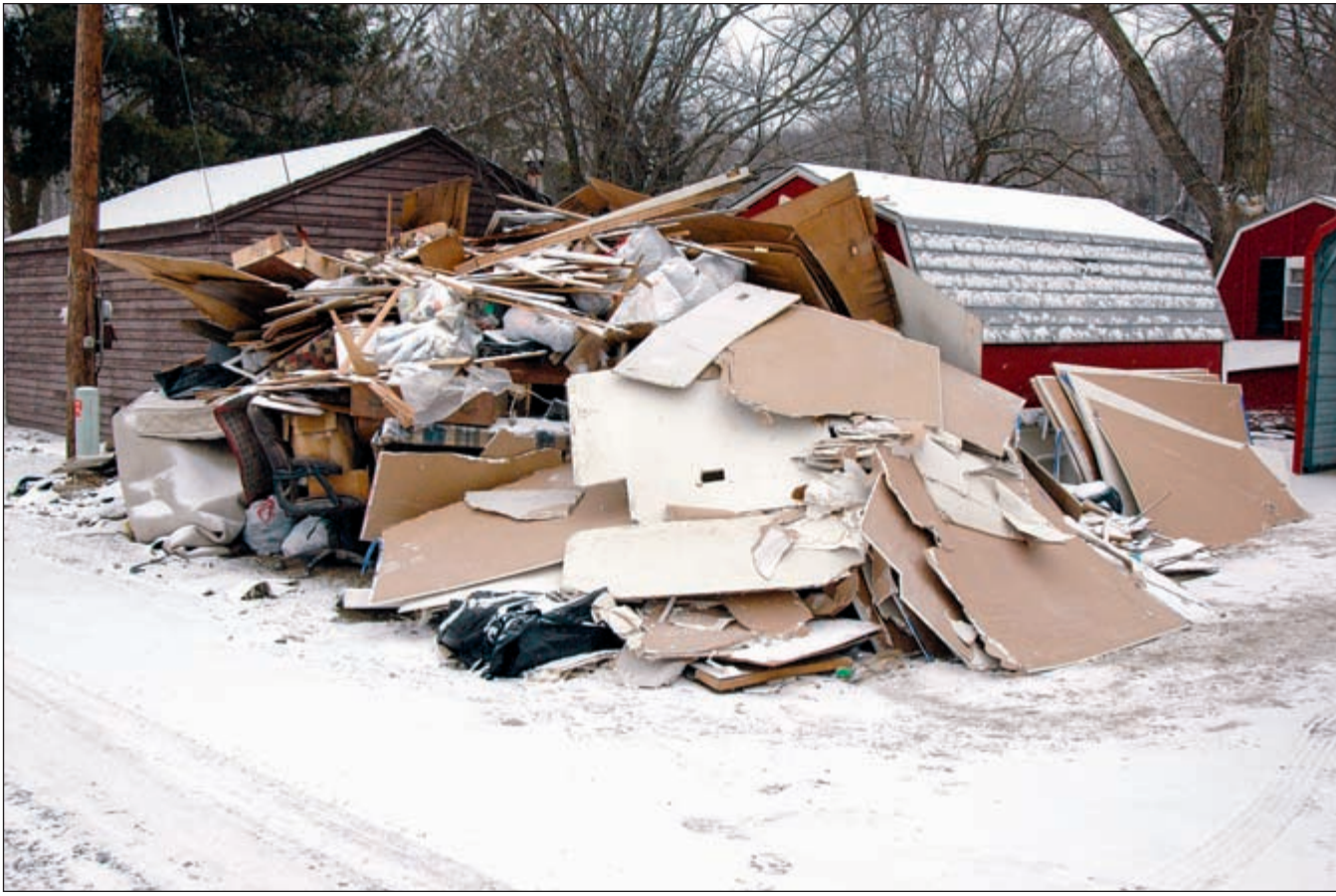
This pile of flood-ravaged debris from the Clark residence in Horseshoe Bend is waiting patiently for county highway to haul it away. Many such piles, some larger and some smaller, line Horseshoe Bend Rd. in Carroll County. Comet photo by Debbie Lowe
