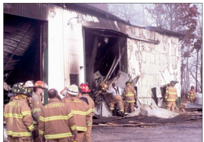
Fire destroyed the Dave Bordner mechanic shop on SR 75.
